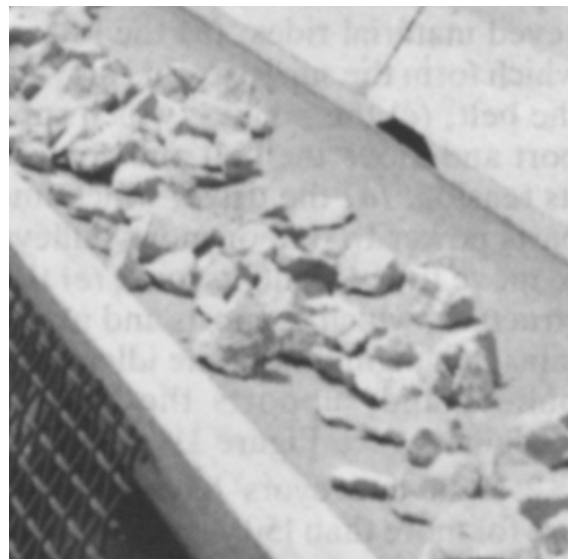
Figure 3. Skirt plates prevent material from falling off conveyors, but also may create nip points at idlers if they prevent belts from lifting freely.
