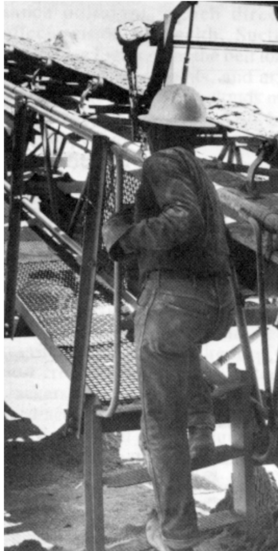
Figure 7. Guards, such as the one shown here, will prevent workers from walking under take-ups.
